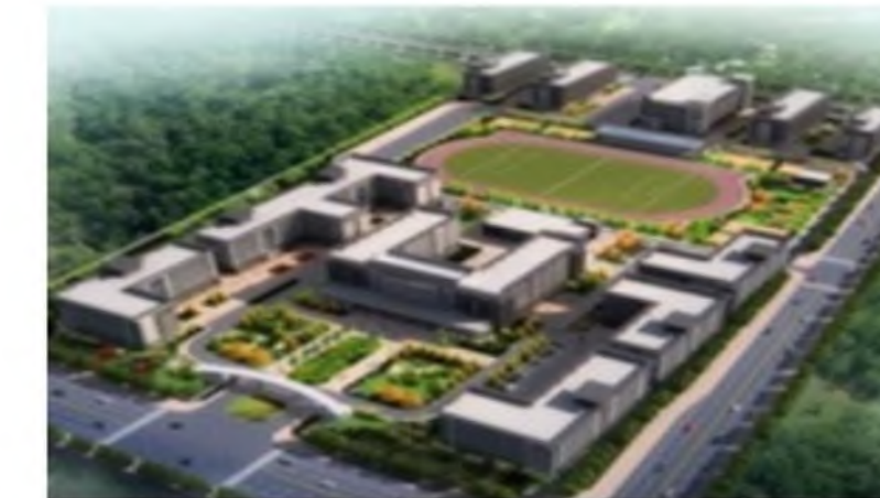
CHINA MOBILE CENTER LUOYANG
